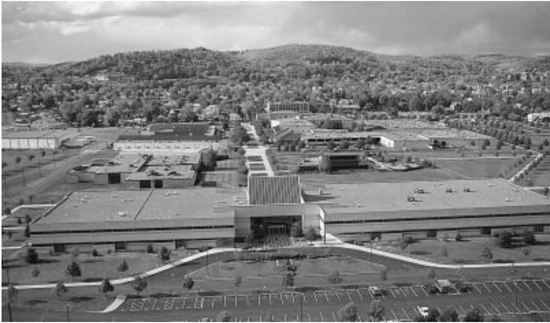
Figure 1. Aerial View of the Applied Technology and Health Sciences Building
